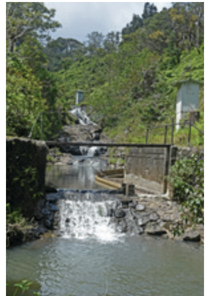
Removed diversion on Honopou Stream, Maui to allow passage of native stream fauna. Photo: Dan Polhemus.
