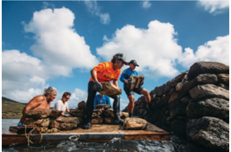
Volunteers at He'eia Fishpond helping to fill in a restored section of kuapā (fishpond wall). Photo: Mark Lee.
